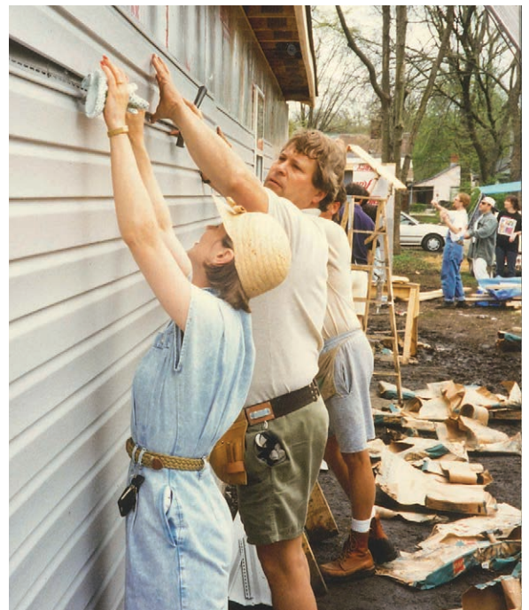
Habitat for Humanity build
