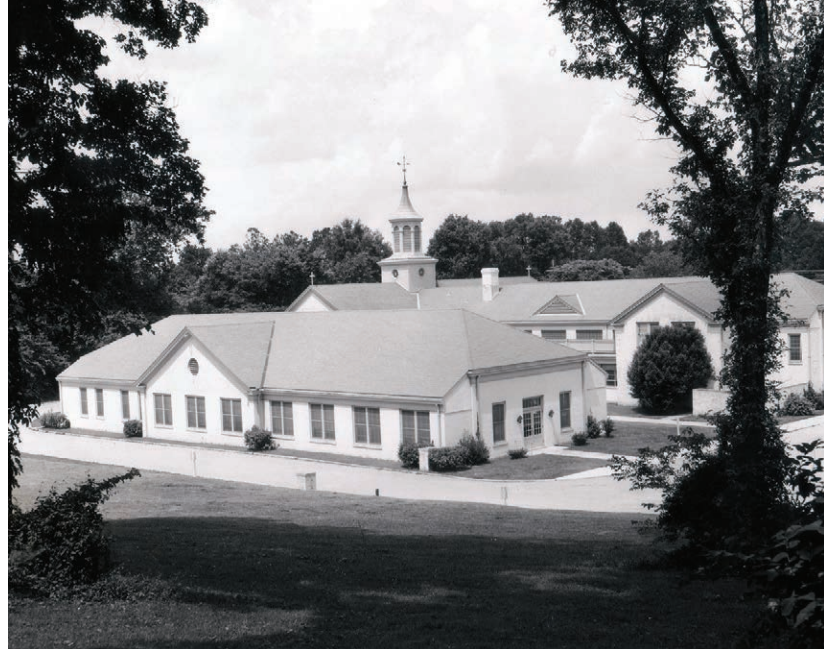
Church exterior after Sunday school addition, 1954
