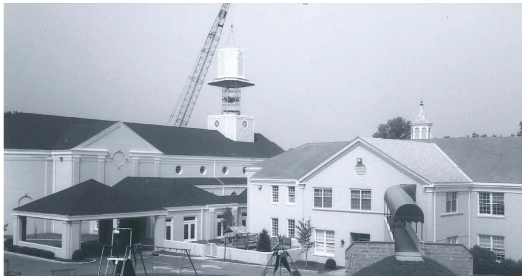
Bell installation and steeple construction, 1987
